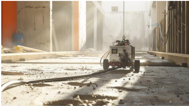
The study looked at how various electrician tasks could be automated - such as cable pulling. Image: AI generated
