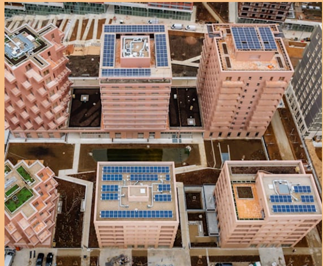
During the Olympics, a photovoltaic carport, over nearly 1,000m 2 , was set up at the bus station and supplied the international delegations' reception centre with self-generated electricity.
