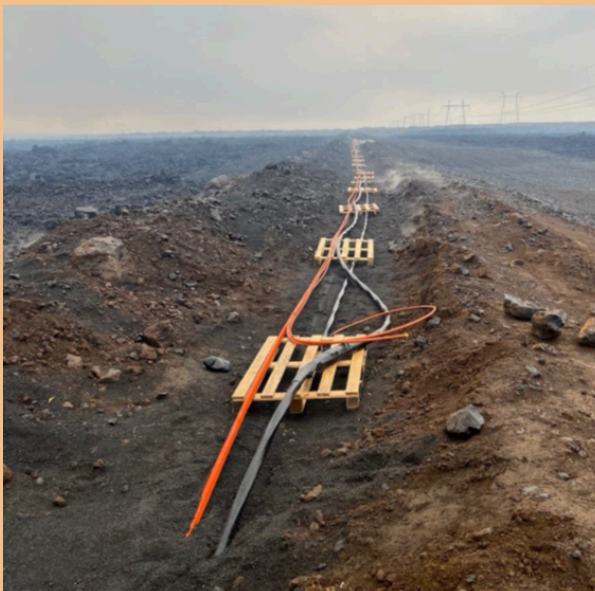
Repairing the fibre optic network in Grindavík, Iceland (courtesy of SART ).
